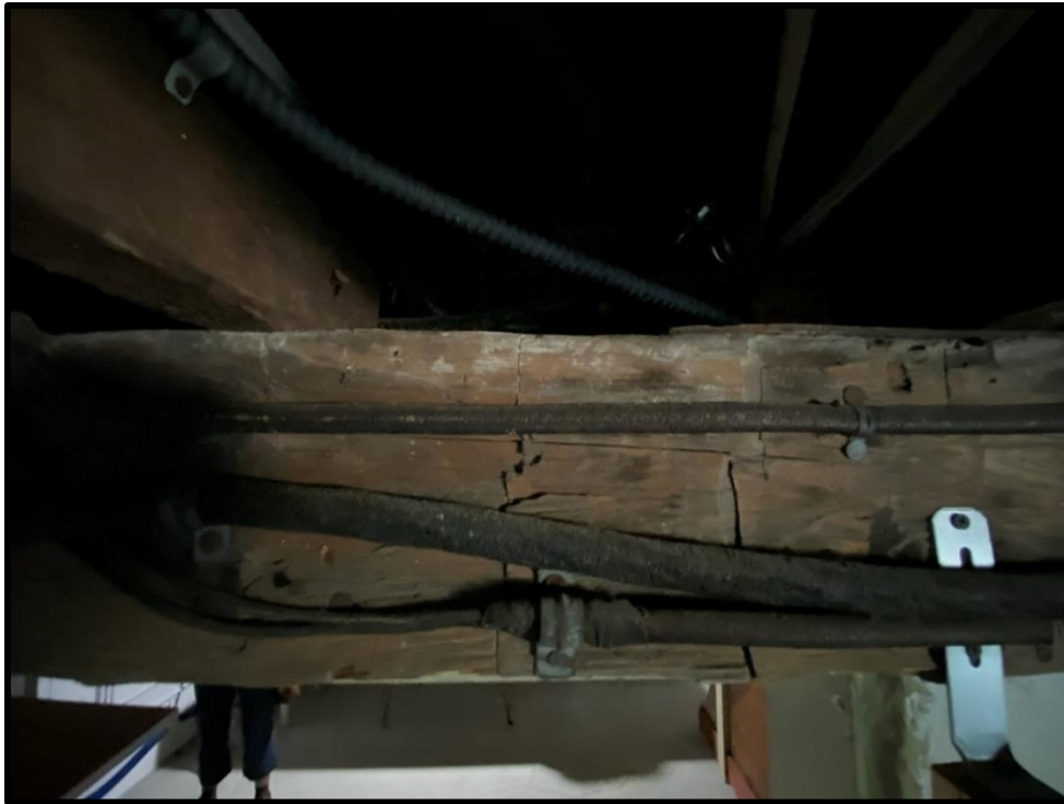
Image 53: Detail of Re-Purposed Timber Beam in Basement – Broadaxe Marks Visible (Photo taken August 31, 2021)
