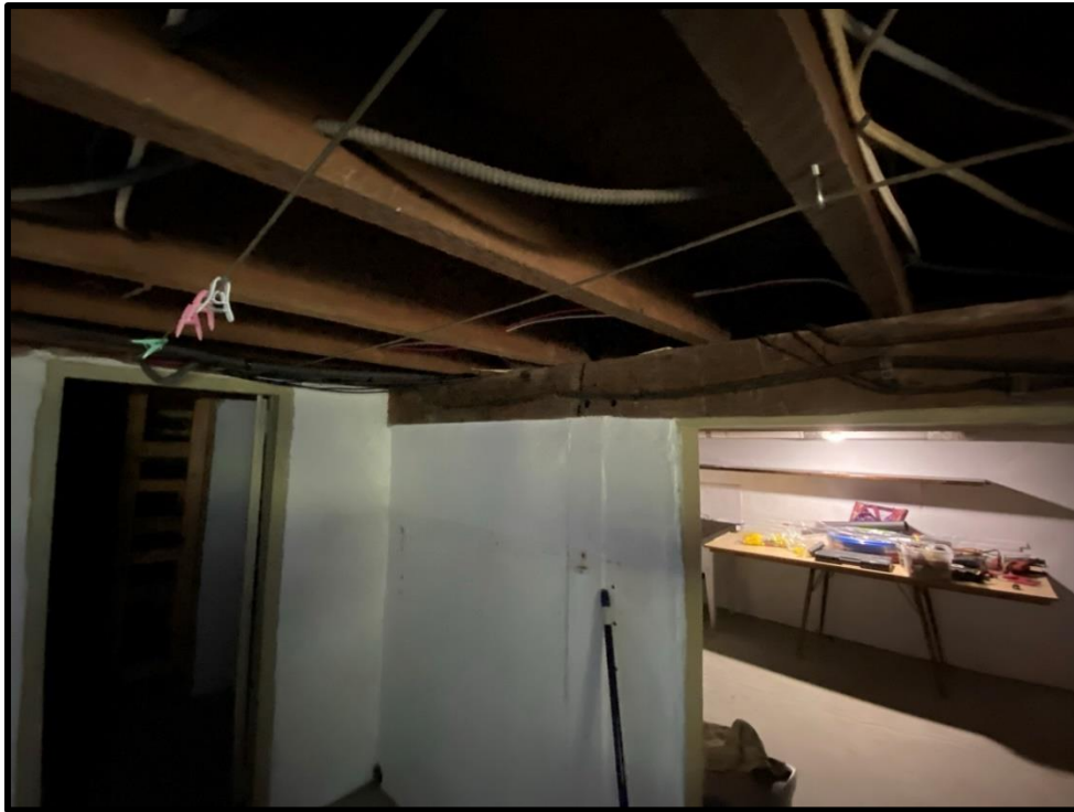
Image 51: View of Re-Purposed Timber Beam in Basement (Photo taken August 31, 2021)
