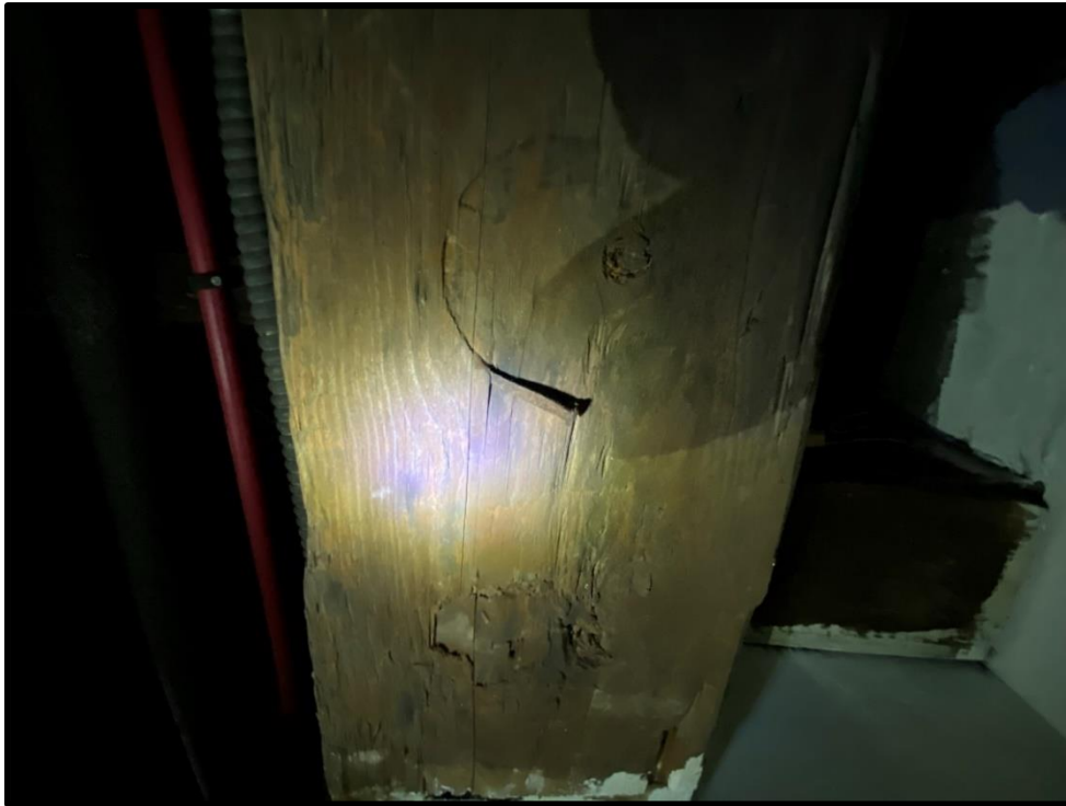
Image 55: Detail of Re-Purposed Timber Beam in Basement – Cut Nail Visible at Centre (Photo taken August 31, 2021)
