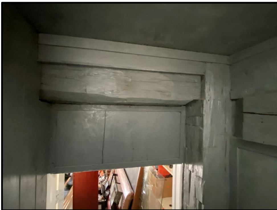
Image 70: Hand Hewn Timbers Connected with Mortice and Tenon Joinery (Photo taken August 31, 2021)
