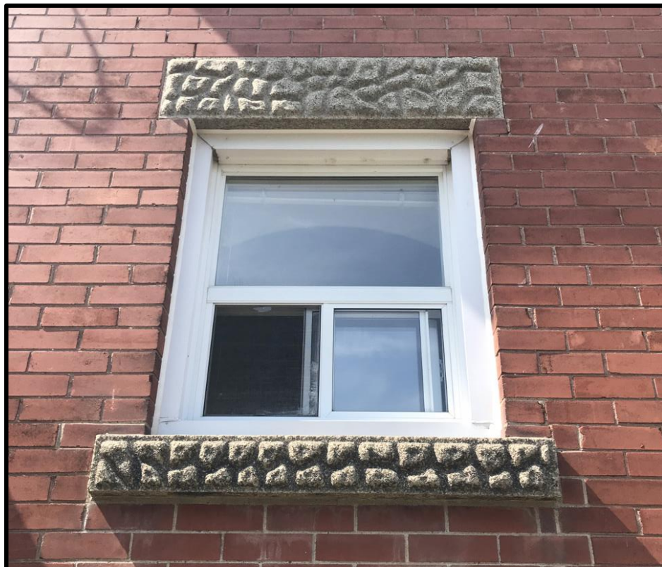
Image 10: Residence – Detail of Window Lintel and Sill with Vermiculated Rustication (Photo taken August 31, 2021; Facing Northwest)
