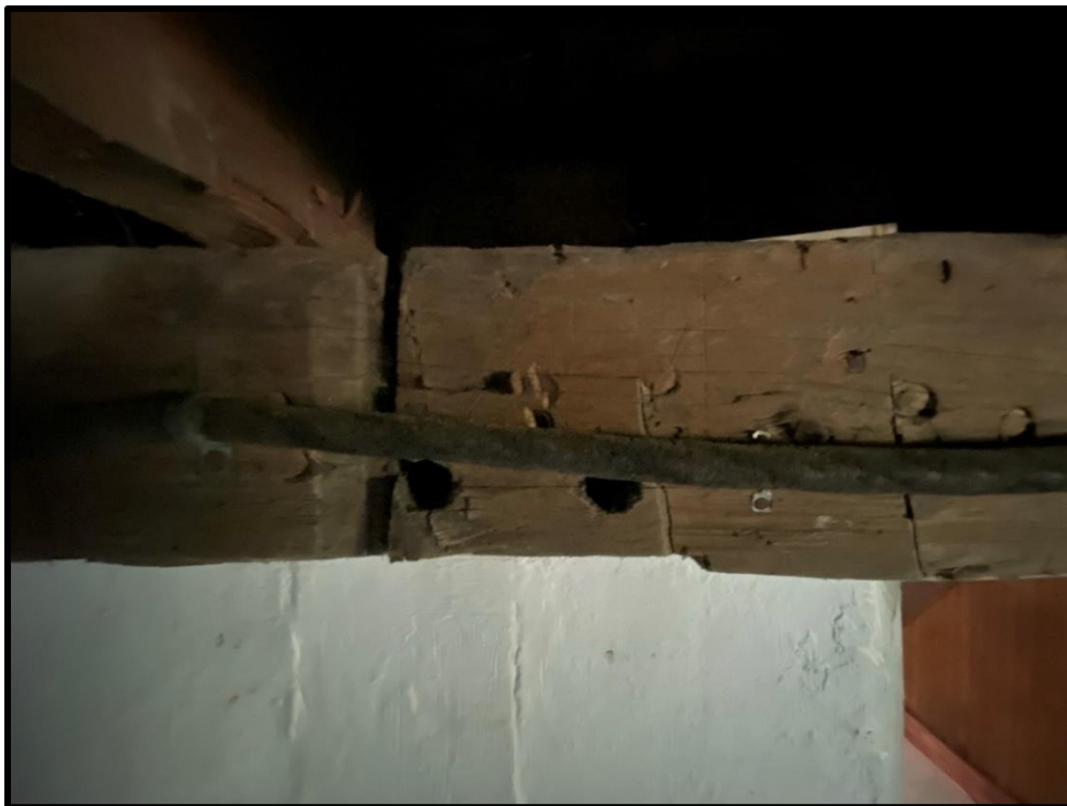
Image 52: Detail of Re-Purposed Timber Beam in Basement – Broadaxe marks and Holes for Wooden Dowels Visible (Photo taken August 31, 2021)
