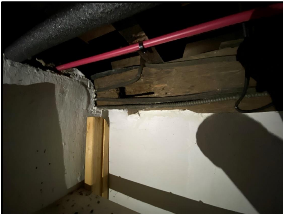
Image 54: Detail of Re-Purposed Timber Beam in Basement – Mortice from Former Mortice and Tenon Joint Visible at Centre (Photo taken August 31, 2021)
