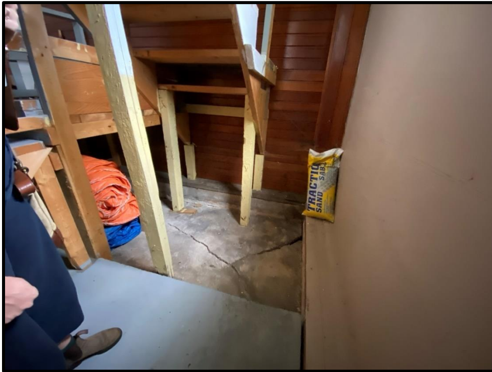
Image 85: Area Underneath Staircase Showing Poured Concrete Floor (Photo taken August 31, 2021)
