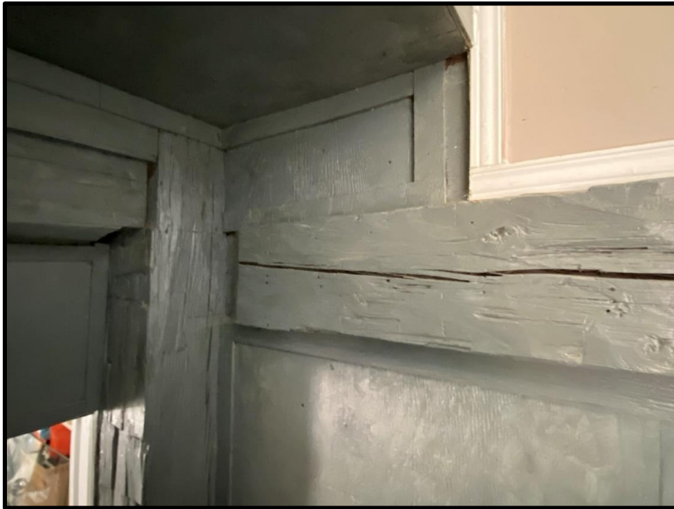
Image 71: Hand Hewn Timbers Connected with Mortice and Tenon Joinery (Photo taken August 31, 2021)
