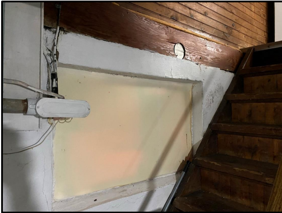
Image 45: View of Covered Basement Window/Parged Foundation (Photo taken August 31, 2021)
