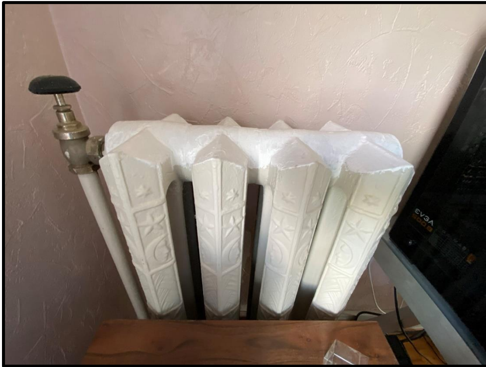
Image 67: Cast Iron Radiator in Second Storey Bedroom (Photo taken August 31, 2021)
