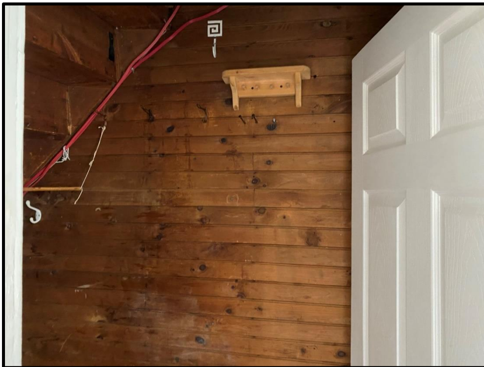
Image 44: Beadboard Cladding in Basement Stairs (Photo taken August 31, 2021)
