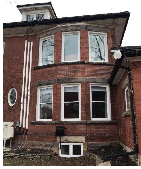
Figure 18: 76 Bower Street, side elevation detail showing projecting bay with flat-headed window openings at the first and second storey with stone sills and lintels (Town of Halton Hills 2022)
