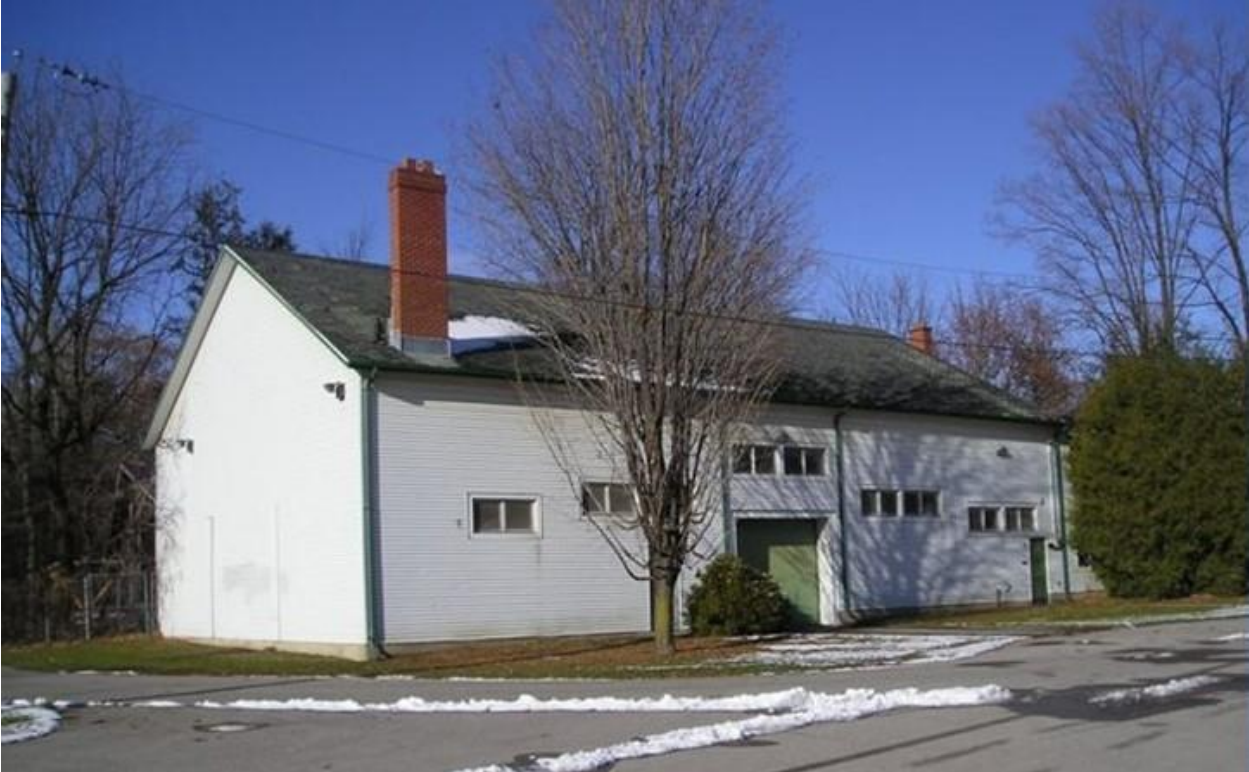
Figure 11: The Armoury in 2009 prior to the renovations. Photo Courtesy of Globe Productions
