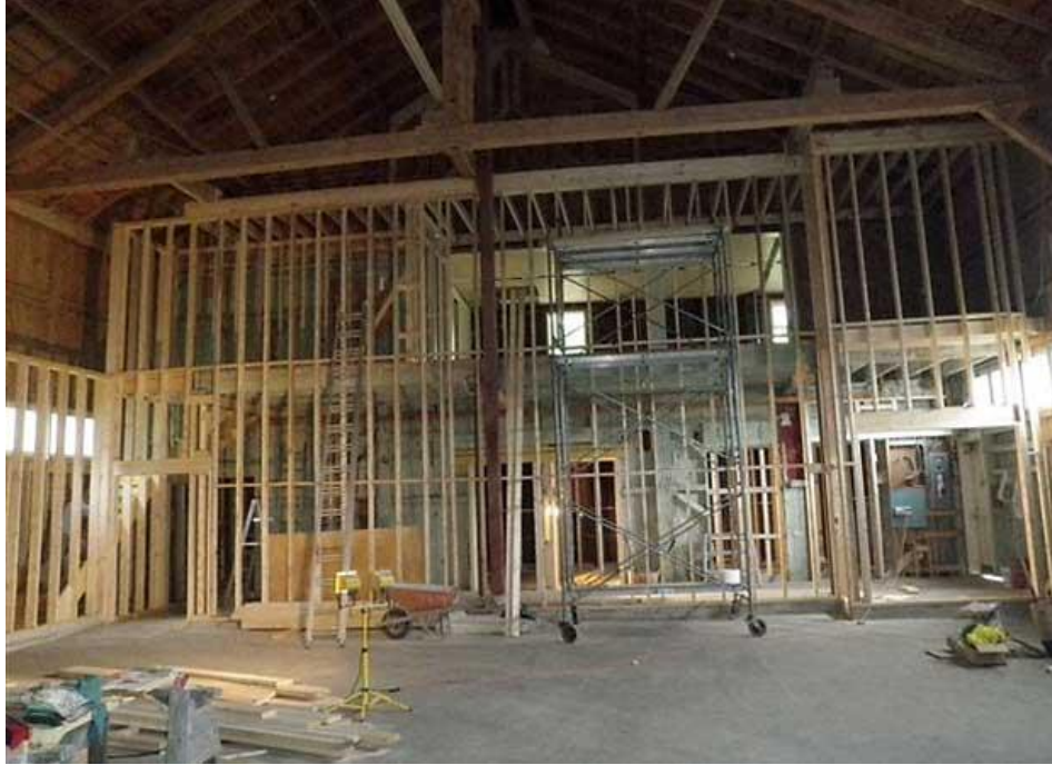
Figure 16: Interior Renovations, including the installation of new walls and stairs for new offices and second floor access. Date between 2010-2015. Image courtesy of Georgetown ON Magazine (georgetownon.ca)
