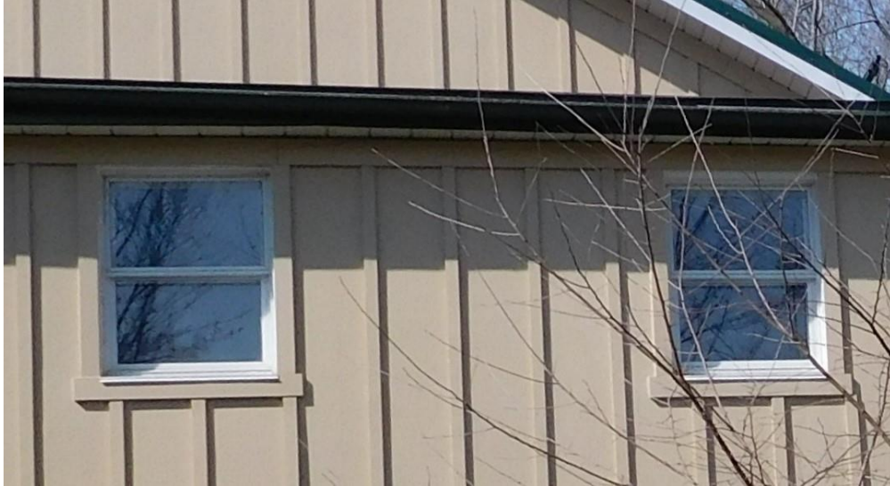
Figure 42: Double Hung Windows can be found on the northeast elevation of the Armoury building. (Town of Halton Hills 2022)
