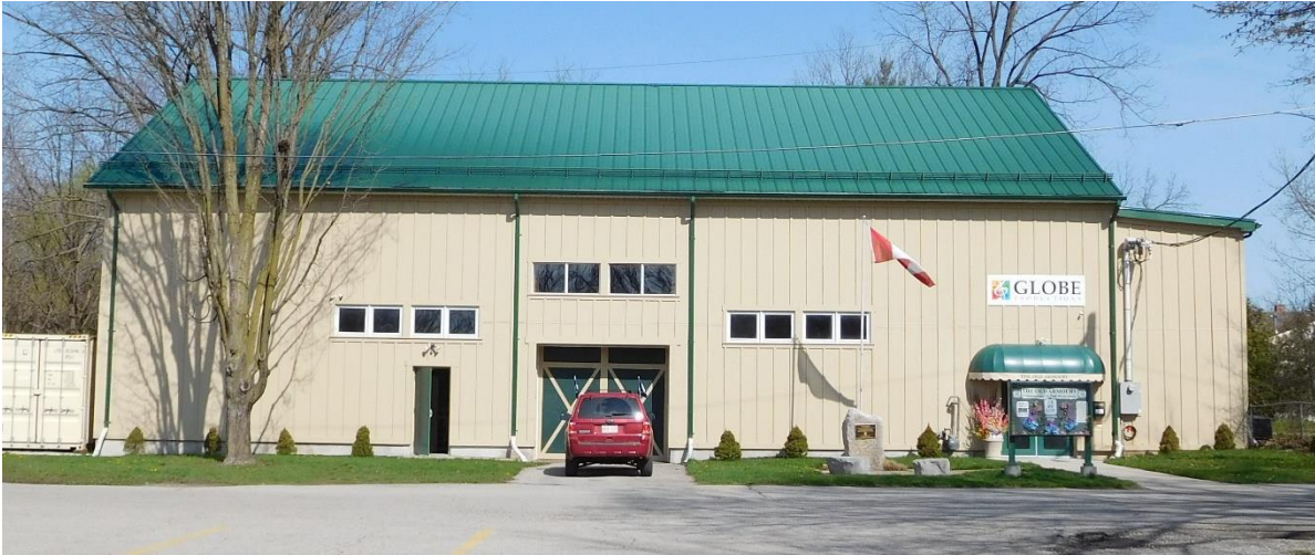
Figure 29: Front (Southeast Elevation) of the structure facing the Fairgrounds parking lot
