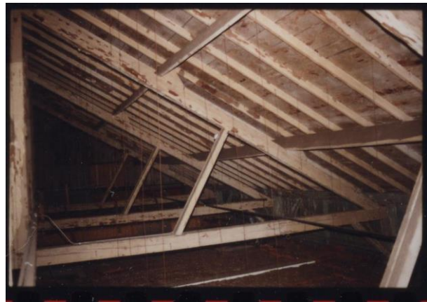
Figure 44: Photo of the roof trusses' structure. (EHS12554)
