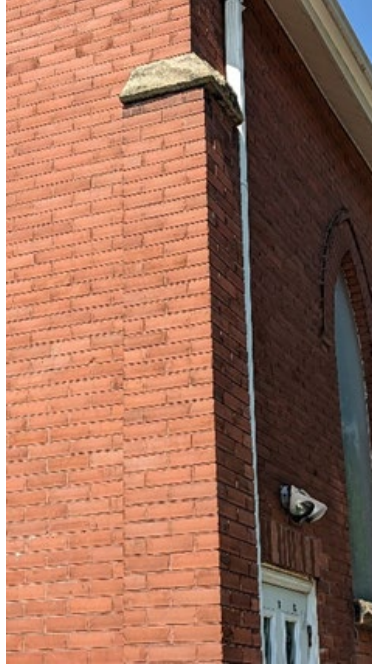
Figure 18: South-west corner buttress (J.M. Rowe June 2023)
