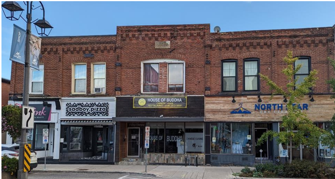
Figure 19: Roe Block at 49-57 Main Street South (John Mark Rowe 2023)
