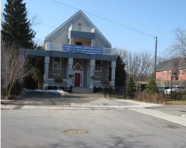
Figure 22: Former Wesleyan Methodist Church, c.2010 (EHS 21148)
