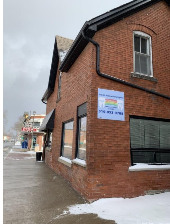
Figure 22: Northwest corner of 46 Mill Street East (Town of Halton Hills 2023)
