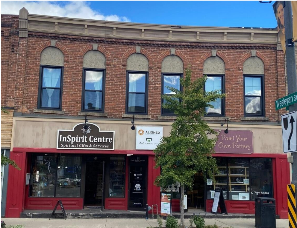
Figure 26: Front (west) elevation of the existing two-storey building (Town of Halton Hills 2023)
