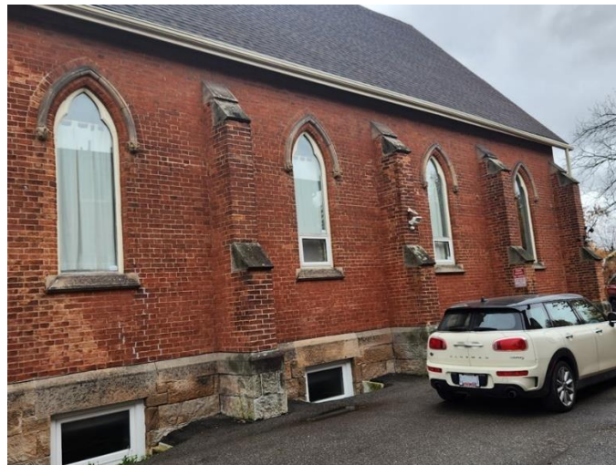
Figure 34: Partial northwest elevation of First Baptist Church (Town of Halton Hills 2023)
