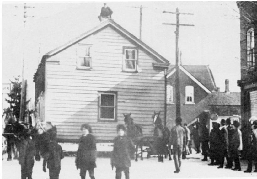
Figure 9: Moving Ransom Adams's House along Mill Street; the subject building is shown to the right of the house being moved, c.1905 (Courtesy of Vintage Acton)
