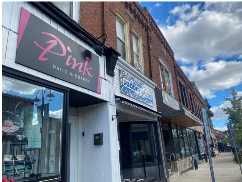
Figure 21: Looking along the front elevation of the subject building (Town of Halton Hills 2023)
