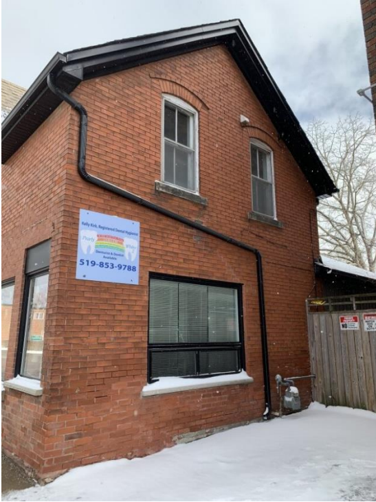
Figure 21: Side (southwest) elevation of 46 Mill Street East (Town of Halton Hills 2023)
