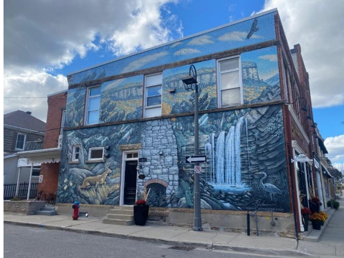
Figure 17: Side (southeast) elevation of 50-52 Main Street South (Town of Halton Hills 2023)
