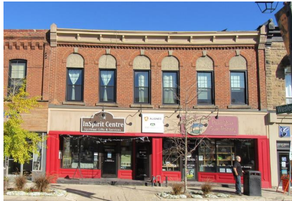
Figure 23: Armour Block in 2022. EHS28490
