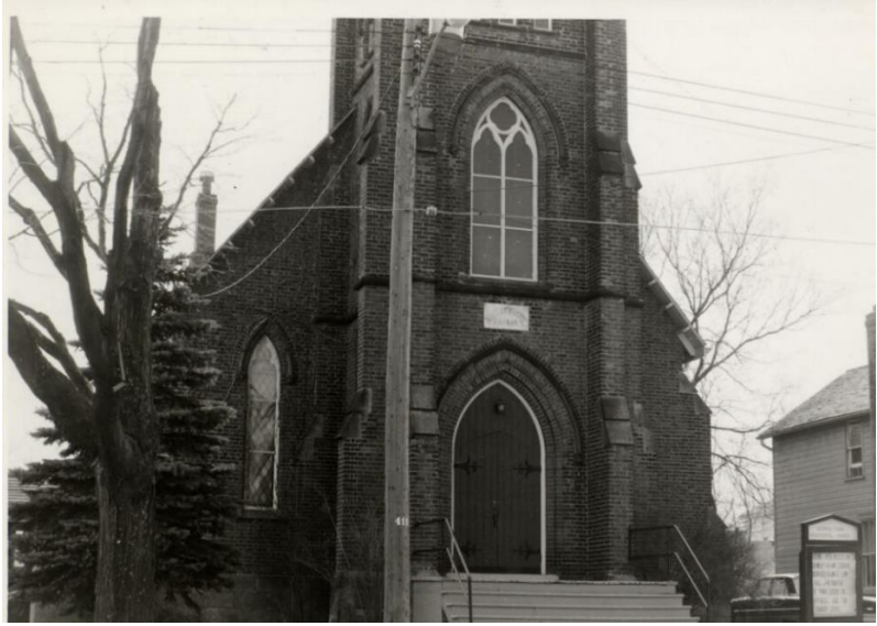
Figure 21: First Baptist Church, c.1973 (EHS 13378)
