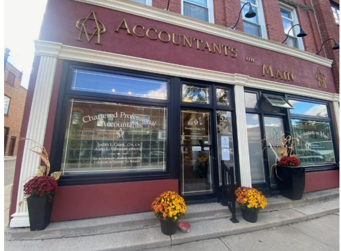
Figure 16: Detail of the front elevation of the existing building at 50-52 Main Street South (Town of Halton Hills)
