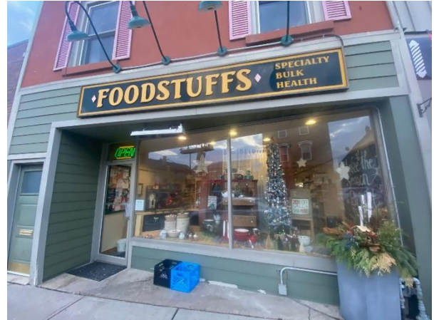
Figure 33: Detail of the front (west) elevation of the existing building (Town of Halton Hills 2023)
