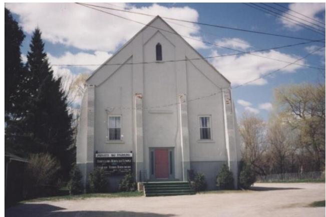
Figure 21: Former Wesleyan Methodist Church, c.1995 (EHS 16805)
