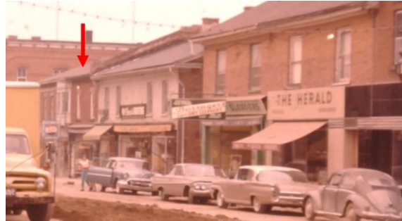
Figure 22: Barclay's Block shown to the left c.1961; the existing portion of Barclay's Block is identified with an arrow (EHS 18401) (detail);
