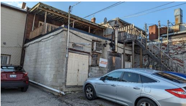
Figure 23: Rear of #55 and 57 Main Street South, showing the 1946 addition in 2023 (John Mark Rowe 2023)
