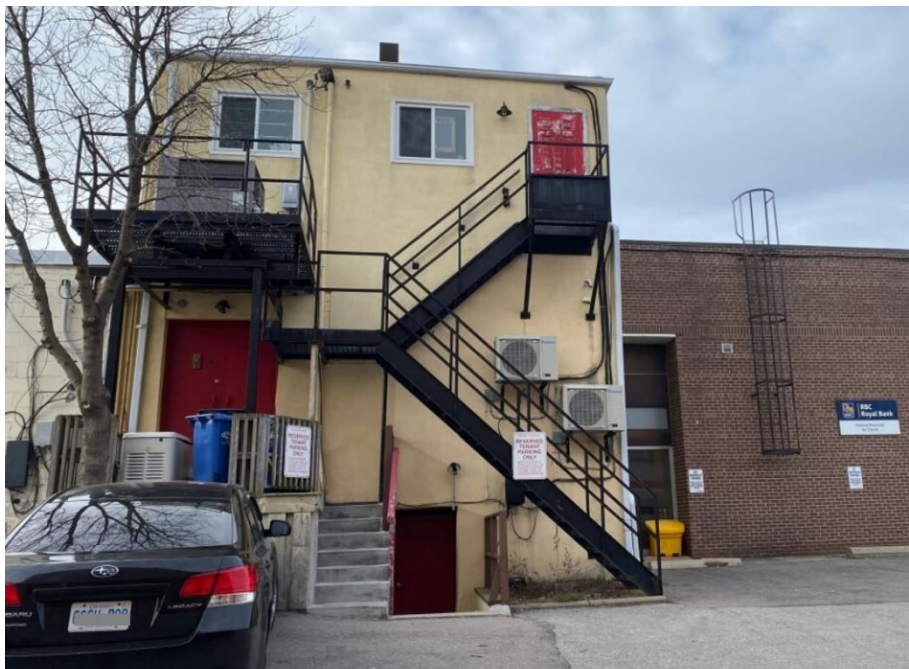
Figure 34: Rear elevation of the existing building from within the municipal parking lot (Town of Halton Hills 2023)
