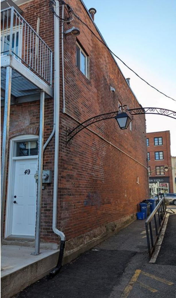
Figure 25: North alley wall in 2023. J.M. Rowe photo
