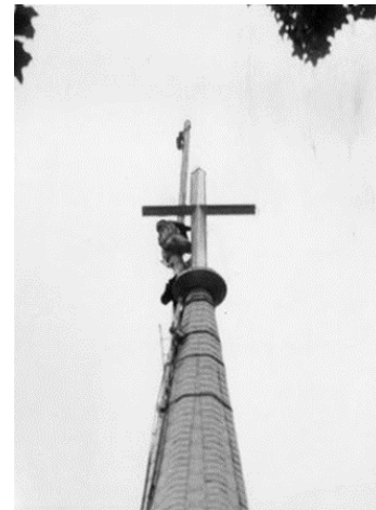
Figure 19: New Hamburg steeplejack Michael Creane secures ten-foot-high gold cross in place atop the First Baptist Church steeple, c. 1961 (EHS 04768)
