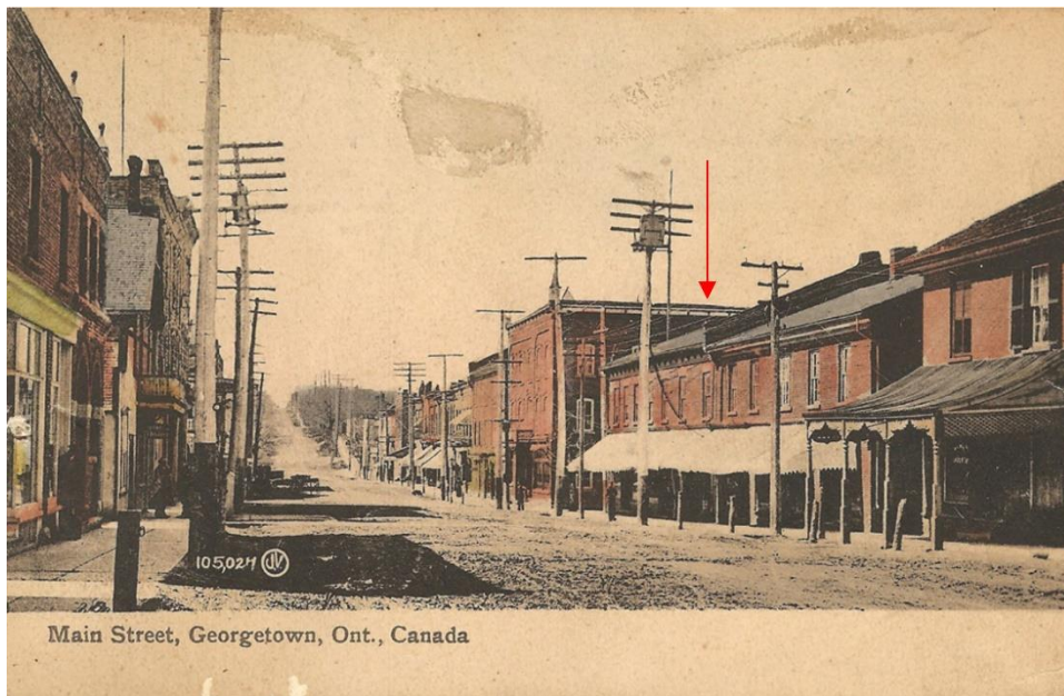
Figure 10: Main Street South, looking north; the existing portion of Barclay's Block is identified with an arrow (EHS 21524)
