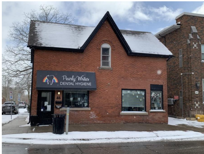
Figure 18: Front (northwest) elevation of 46 Mill Street East (Town of Halton Hills 2023)
