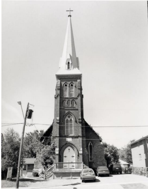
Figure 22: First Baptist Church, c.1980 (EHS 13021)
