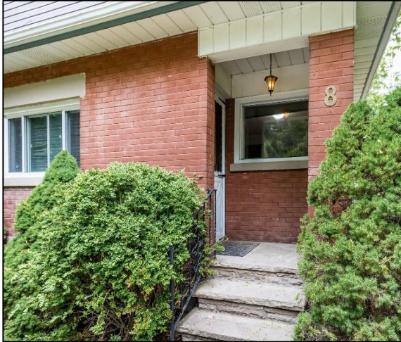
Figure 18: Recessed porch located on the front elevation (Tours4Listing 2023)
