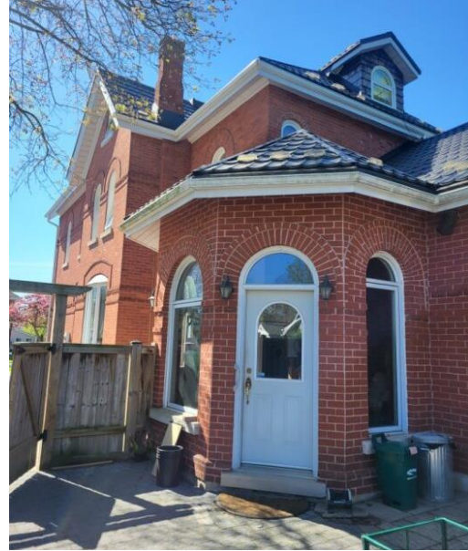
Figure 23: Partial side (northeast) elevation as seen from the rear yard
