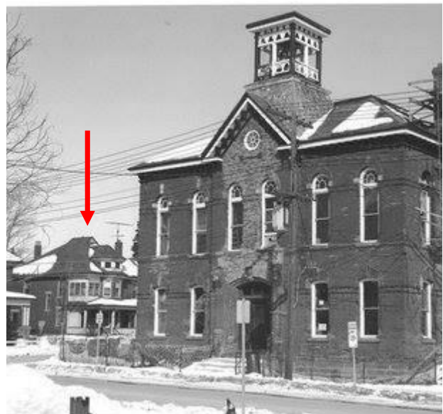
Figure 21: Town Hall with the subject property in the background, c.1984 (EHS 13762)
