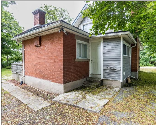
Figure 24: Rear (northeast) elevation of the existing dwelling, and rear addition (Tours4Listing 2023)
