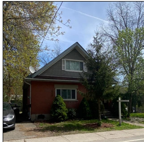
Figure 17: Front (southwest) elevation of the existing dwelling (Town of Halton Hills 2024)
