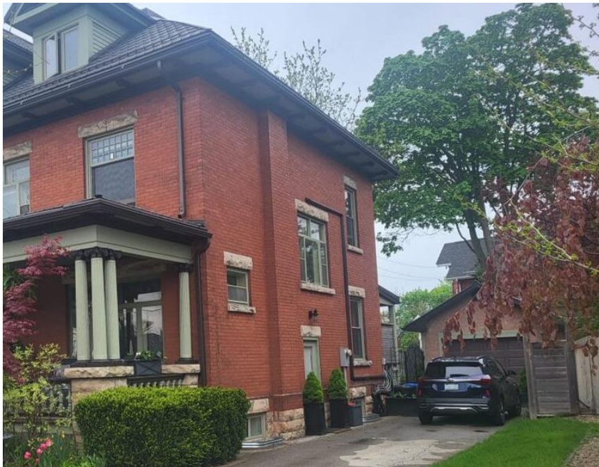
Figure 29: Side (northeast) elevation of the existing building at 29 Bower Street (Town of Halton Hills 2024)
