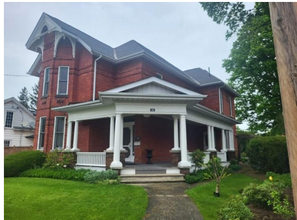
Figure 21: Southwest corner of the existing building at 39 Willow Street North (Town of Halton Hills 2024)
