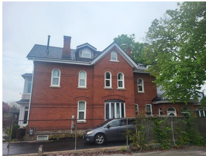
Figure 24: Side (northeast) elevation (Town of Halton Hills 2024)
