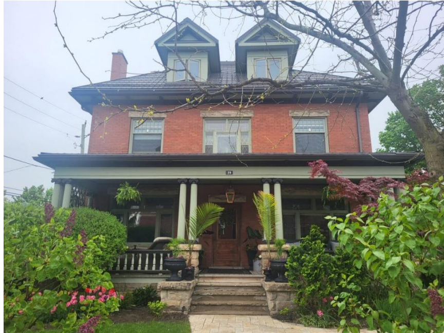
Figure 28: Front (southeast) elevation of the existing building at 29 Bower Street (Town of Halton Hills 2024)
