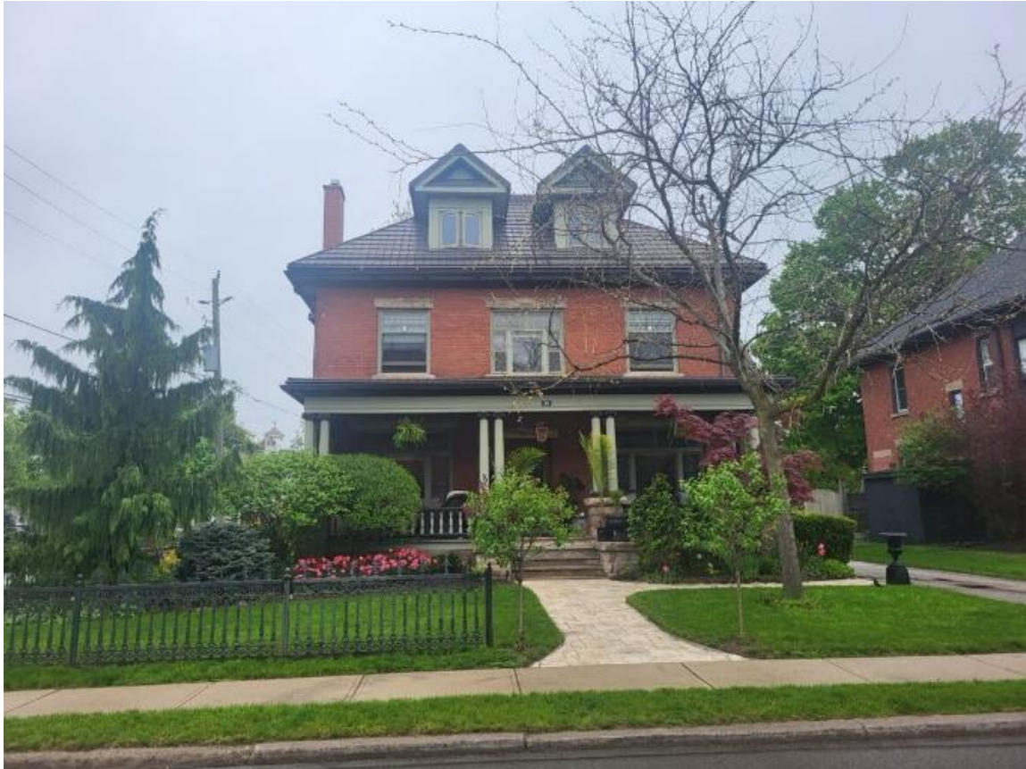
Figure 27: Looking towards the front elevation from Bower Street (Town of Halton Hills 2024)
