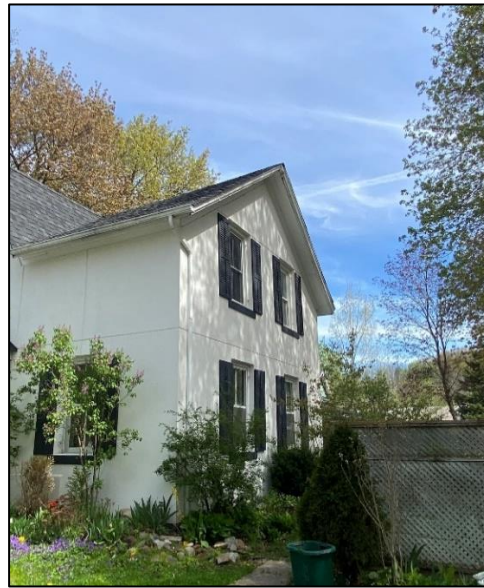
Figure 21: South corner of the existing dwelling (Town of Halton Hills 2024)
