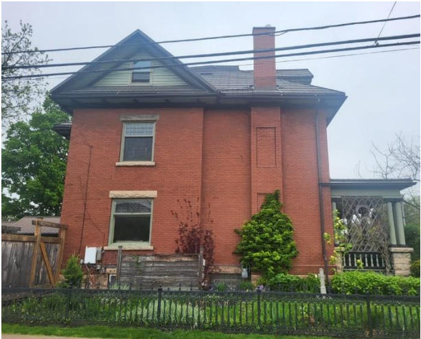
Figure 30: Side (southwest) elevation of the existing building at 29 Bower Street (Town of Halton Hills 2024)
