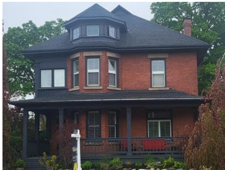
Figure 22: The front (southeast) elevation of the existing residence at 35 Bower Street (Town of Halton Hills 2024)
