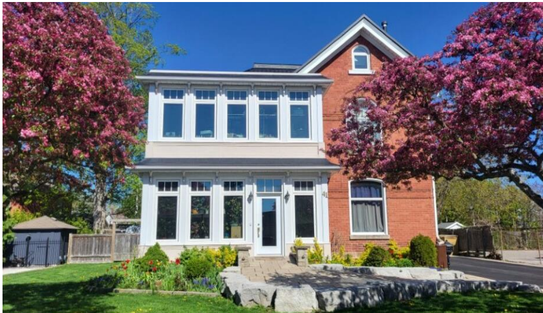
Figure 21: Front (southeast) elevation (Town of Halton Hills 2024)
