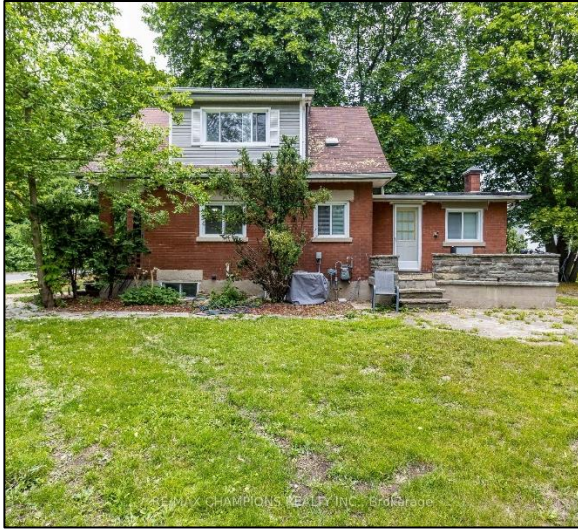
Figure 22: Side (southeast) elevation of the existing dwelling (Tours4Listing 2023)
