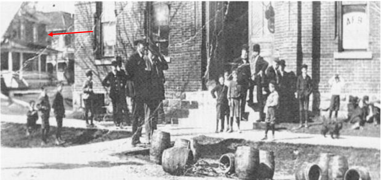
Figure 15: Contraband beer from the Dominion Hotel was poured down the gutter in front of Town Hall, c.1911. The subject property is identified with a red arrow in the background (A.T. Brown/Dills Collection - Vintage Acton)
