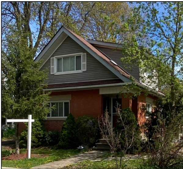
Figure 16: South corner of the existing dwelling (Town of Halton Hills 2024)
