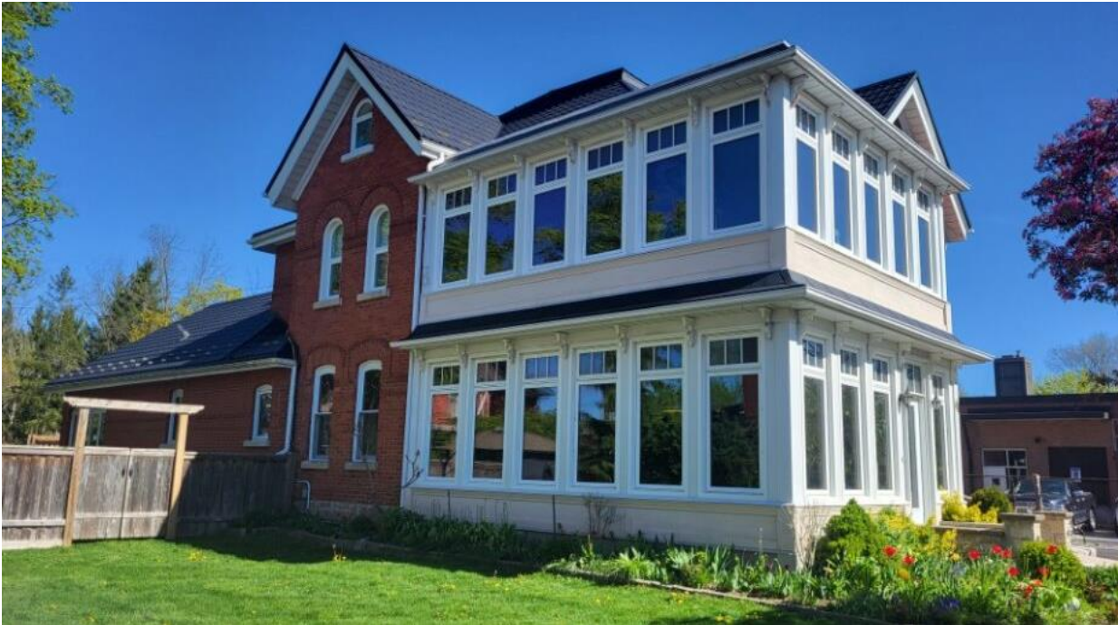
Figure 25: Side (southwest) elevation (Town of Halton Hills 2024)
