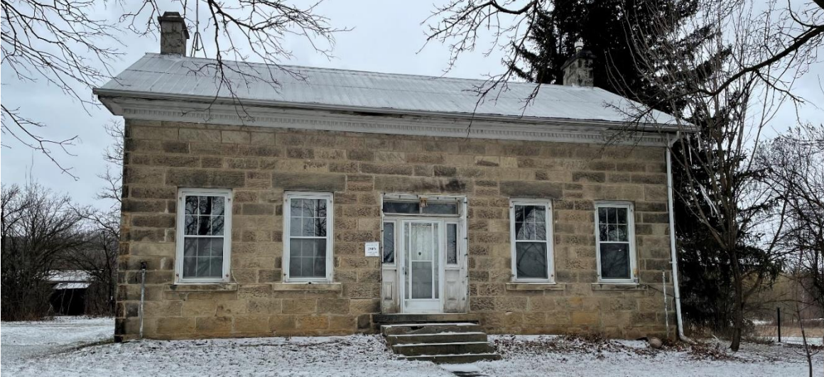
Figure 22: Front (southeast) elevation of the Duncan McCallum House (Town of Halton Hills 2024)
