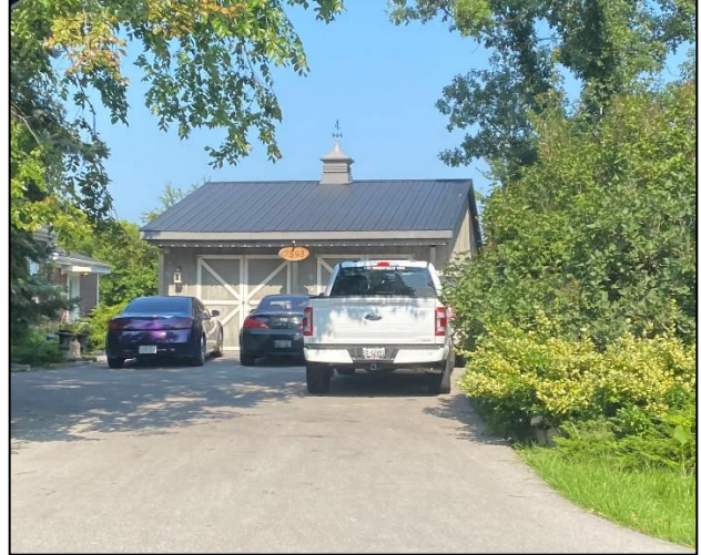
Figure 41: Accessory structure adjacent to subject dwelling (Town of Halton Hills 2024)
