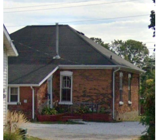
Figure 14: 56 Young Street, rear Elevation. (Town of Halton Hills, 2024)
