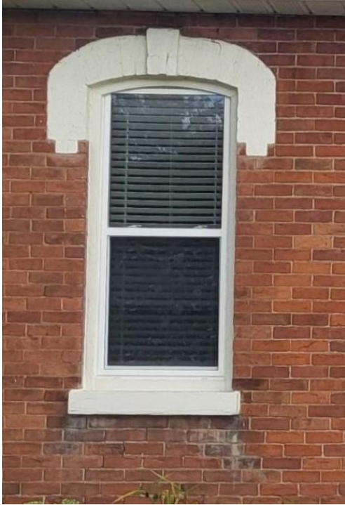
Figure 17: Window Detailing on 23 Young Street. (Town of Halton Hills, 2024)
