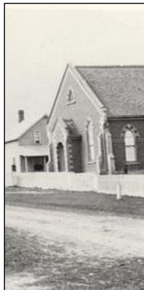
Figure 6: Former Presbyterian Church, Ballinafad, c.1900 (EHS12153)
