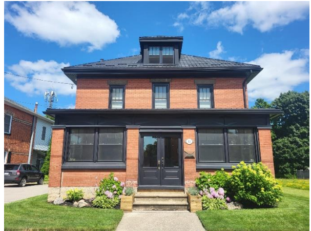
Figure 19: Front (southeast) elevation of the existing building on Bower Street (Town of Halton Hills 2024)
