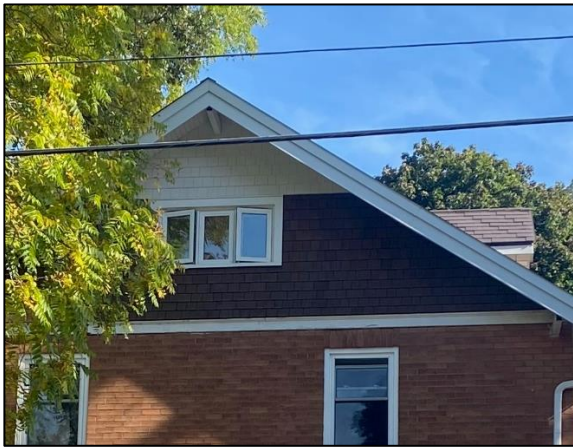
Figure 27: Existing cedar shingles beneath the gable peak, along the front elevation (Town of Halton Hills 2023)
