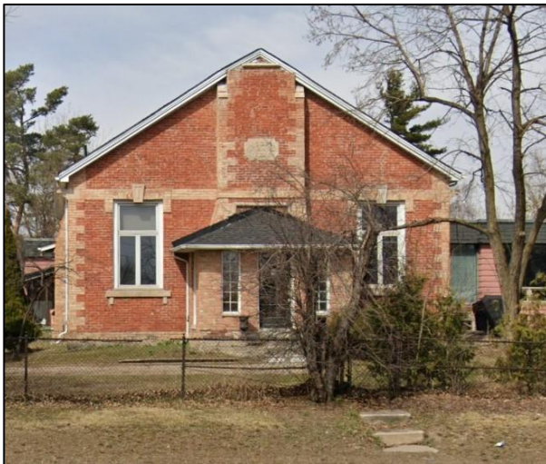
Figure 48: Former Hornby School along Steeles Avenue (Google Streetview, 2021)
