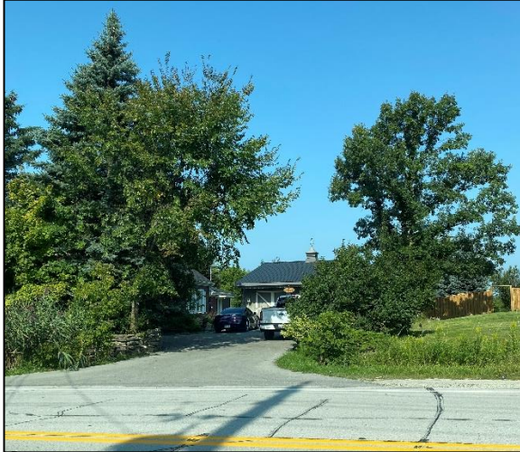
Figure 40: Partial side (northeast) elevation of the subject dwelling (Town of Halton Hills 2024)
