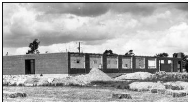
Figure 22: Construction of Pineview School, c. 1963 (EHS06426)
