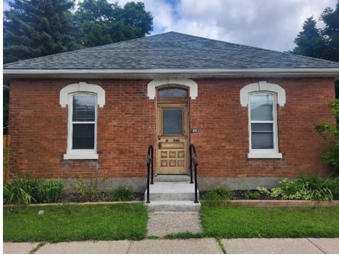
Figure 9: 23 Young Street, Front (South) Elevation (Town of Halton Hills 2024)
