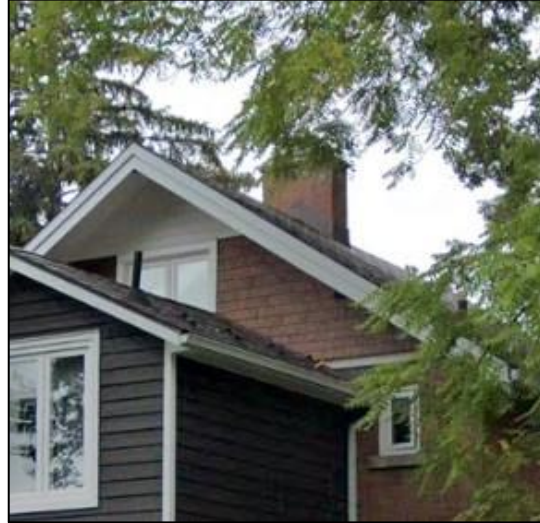
Figure 34: Flat-headed window openings along the remaining original elevation (Google Streetview 2019)
