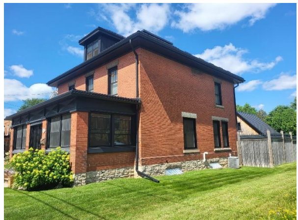
Figure 21: Southwest corner of the existing building at 93 Bower Street, showing the side (northwest) and front (southeast) elevations (Town of Halton Hills 2024)
