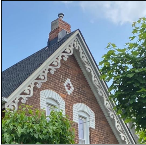
Figure 25: Decorative white lozenge pattern directly above the bay on the front (northwest) elevation (Town of Halton Hills 2024)
