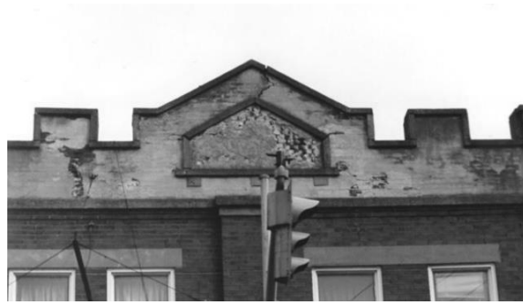
Figure 22: A 1996 photograph of Parapets on Starkman Block constructed in 1922. (EHS 23573)
