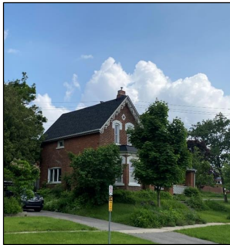
Figure 28: Partial side (northeast) elevation of the existing dwelling (Town of Halton Hills 2024)
