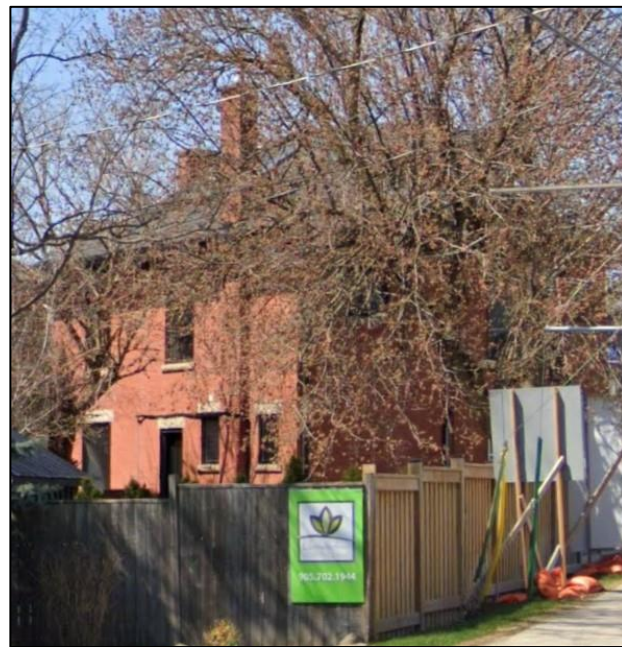
Figure 37: Partial rear (southeast) and side (northeast) elevations presently obscured by vegetation (Google Streetview 2022)
