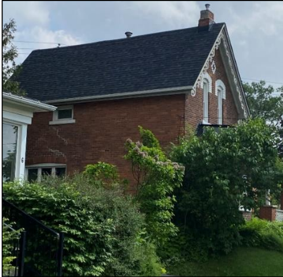
Figure 29: Side (southeast) elevation of the existing dwelling (Town of Halton Hills 2024)
