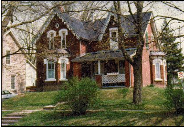
Figure 18: 4 Queen Street c. 1990 (EHS10596)
