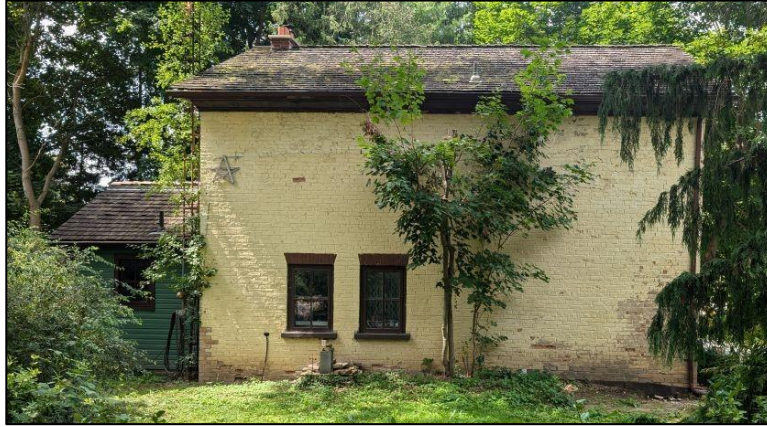
Figure 29: Side (east) elevation of the existing dwelling (John Mark Rowe 2024)
