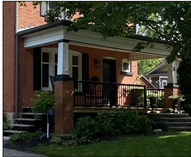
Figure 33: Existing covered wooden porch along the front (southwest) elevation (Town of Halton Hills 2024)
