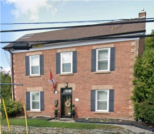
Figure 24: A Georgian Residence at 510 Main Street, Glen Williams. (Google Street View 2023)
