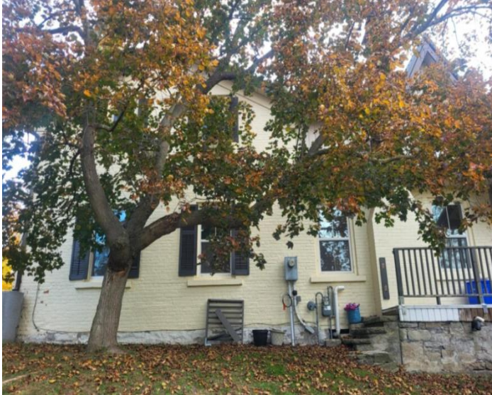
Figure 23: Side (southwest) elevation of the existing building at the subject property, slightly obscured by mature tree (Town of Halton Hills 2024)
