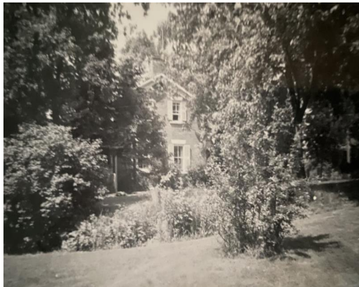
Figure 11: Northeast elevation of 15 Mountain Street in 1961 (Courtesy of Christine Earl 2024)
