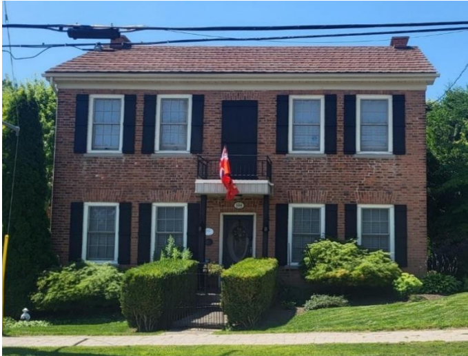
Figure 23: A Georgian Residence at 504 Main Street, Glen Williams. (Town of Halton Hills 2024)
