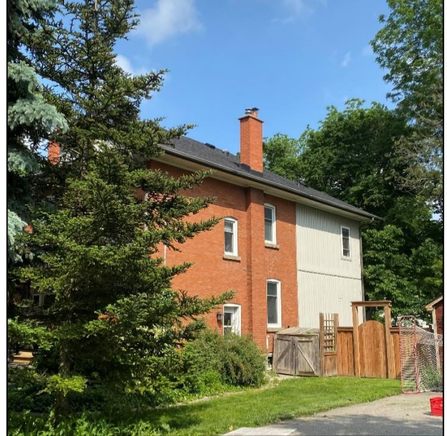
Figure 35: Side (southwest) elevation of the existing dwelling (Town of Halton Hills 2024)
