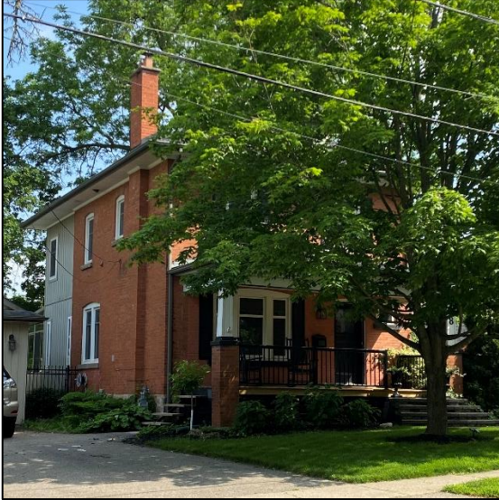
Figure 30: Obscured front (northwest) elevation of the existing dwelling (Town of Halton Hills 2024)
