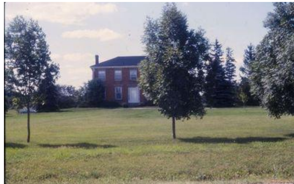
Figure 10: The subject property at 10295 10 Side Road c.1990s (EHS 18312).
