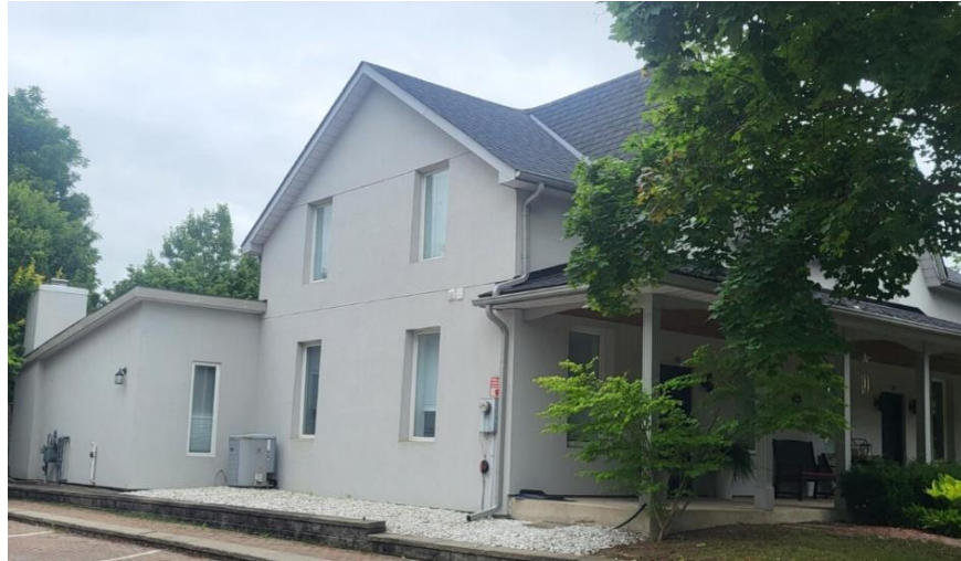
Figure 26: Side (north) elevation of the existing building at 12 & 14 Adamson Street North (Town of Halton Hills 2024)
