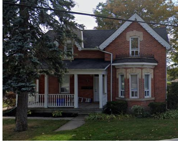
Figure 42: Example of an L-shaped Gothic Revival residence in a town setting in Halton Hills at 67 Young Street, Acton (Town of Halton Hills 2024)
