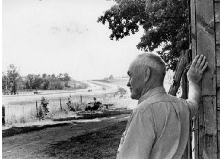
Figure 16: Chisholm observes the development of his land at Lot 5, Concession 6, Nassagaweya for Highway 401. ( The Georgetown Herald , July 7, 1969, p. 5)
