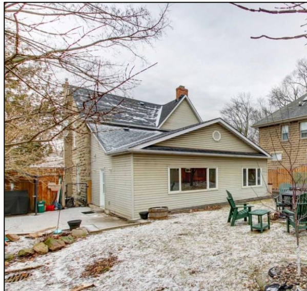
Figure 29: Rear (southeast) elevation featuring the contemporary addition (HouseSigma 2022)
