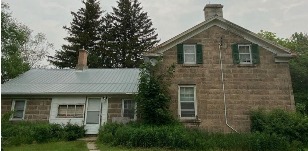
Figure 29: Side (southwest) elevation of the Duncan McCallum House (Courtesy of Avison Young)
