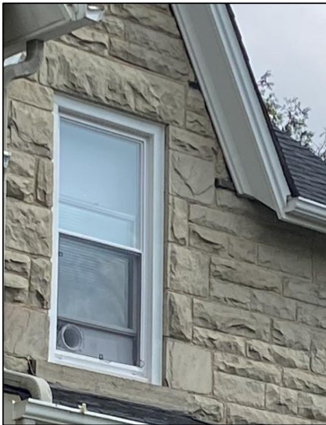
Figure 23: Stone quoining surrounding the existing window openings (Town of Halton Hills 2024)
