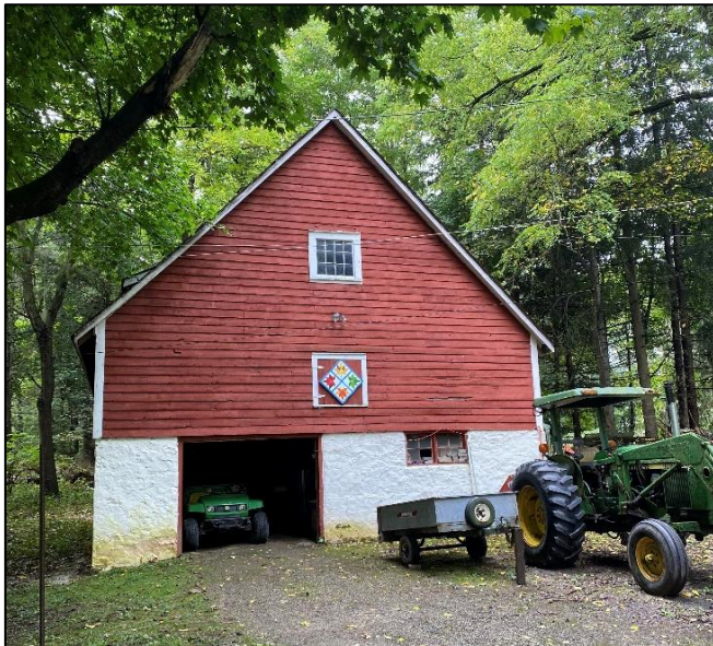
Figure 41: Front (northeast) elevation of the accessory barn structure (Town of Halton Hills 2024)
