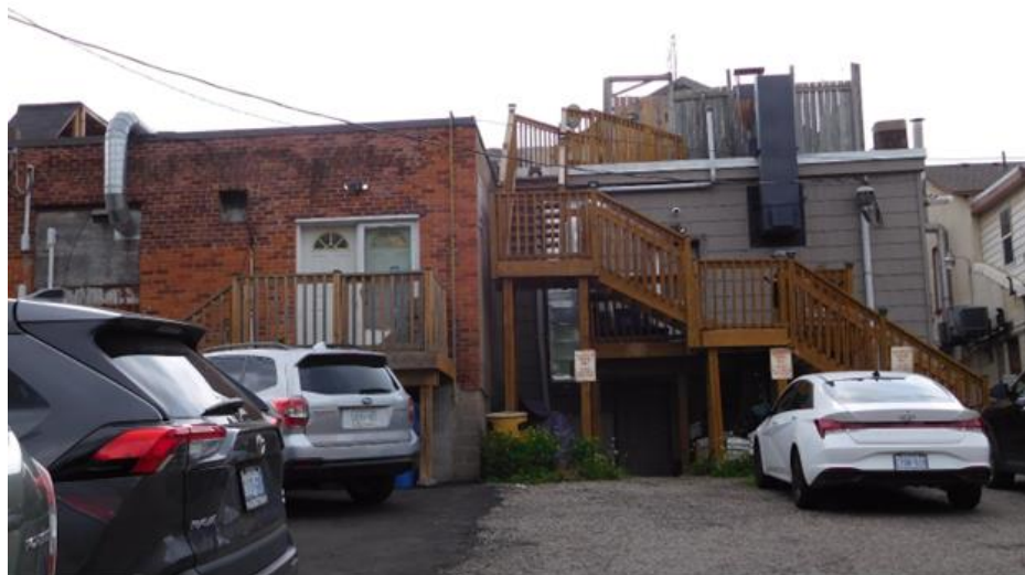
Figure 29: Rear elevation of the existing building, showing rear one-storey additions (Town of Halton Hills 2022)
