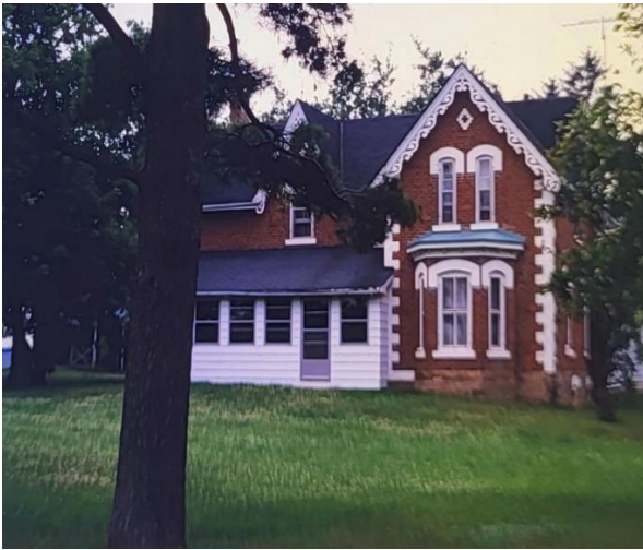
Figure 32: A 1983 photograph of 9709 Fifth Line including a sunroom on the Front Elevation (EHS 18247)
