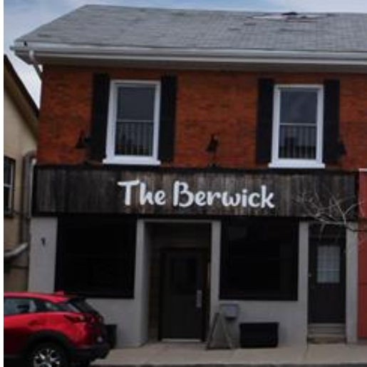
Figure 26: Partial west elevation (Town of Halton Hills, 2022)
