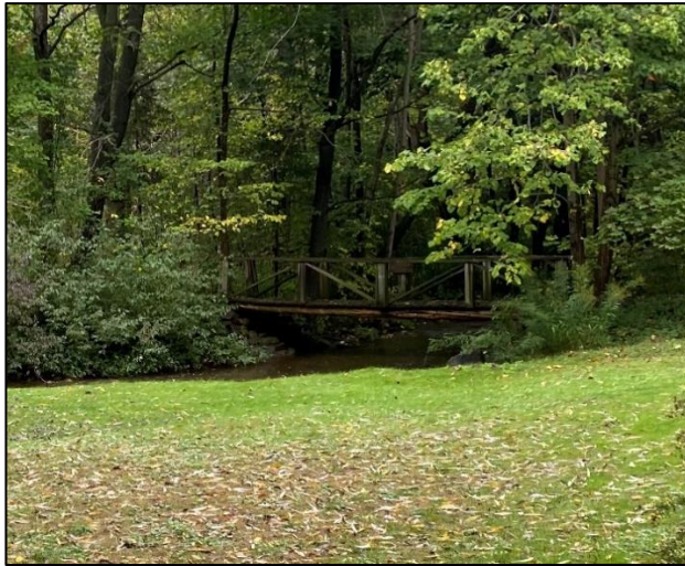
Figure 45: Wooden bridge spanning Silver Creek towards the rear of the property (Town of Halton Hills 2024)
