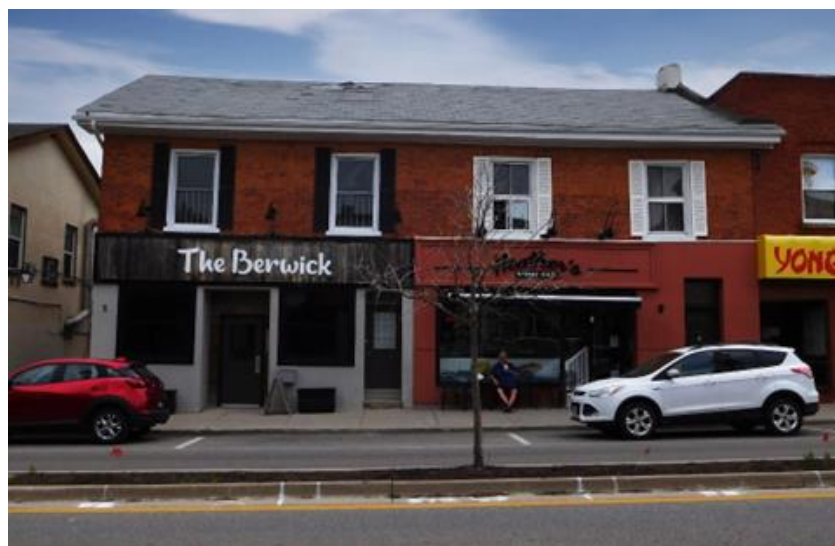
Figure 25: 99-103 Main Street Front (West) Elevation (Town of Halton Hills, 2022)
