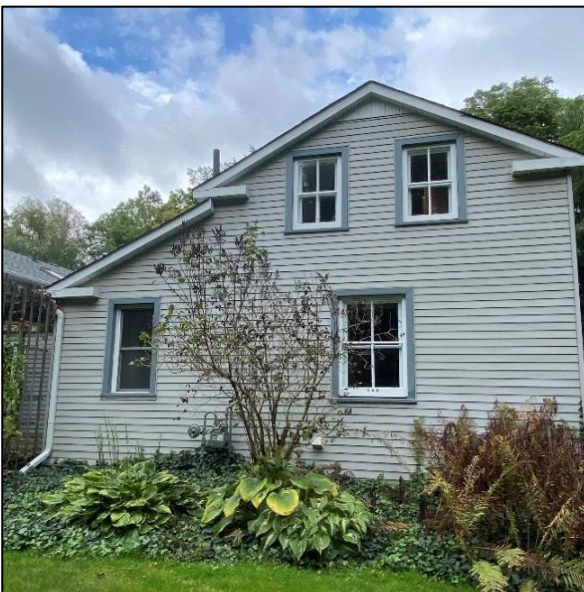
Figure 37: Side (southeast) elevation of the subject dwelling (Town of Halton Hills 2024)
