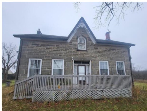
Figure 31: The c.1870s Gothic Revival farmhouse located on Lot 6, Concession 1 at 9401 Dublin Line (Town of Halton Hills 2024)
