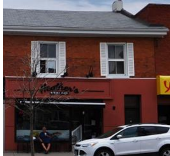
Figure 27: Partial west elevation (Town of Halton Hills, 2022)
