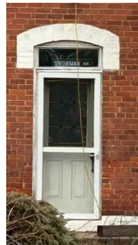
Figure 29: Segmentally arched entrance with painted voussoir and transom window at the first storey (Town of Halton Hills 2024)
