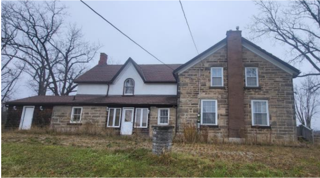
Figure 24: Side (southeast) elevation (Town of Halton Hills 2024)
