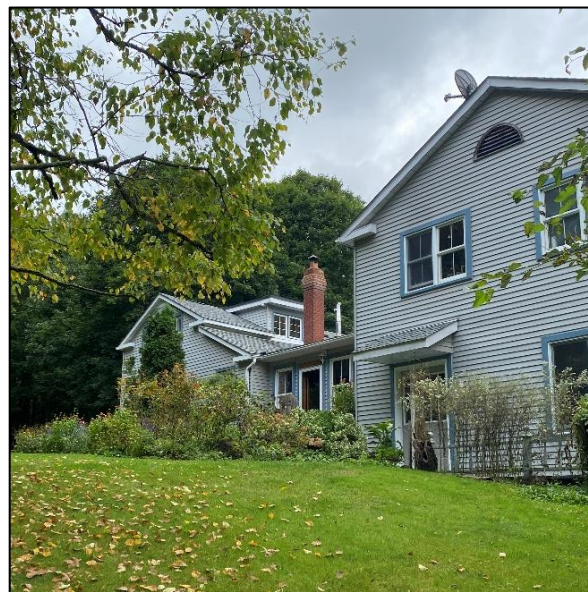
Figure 38: Partial side (northwest) elevation of the subject dwelling, showing the middle and rear additions (Town of Halton Hills 2024)
