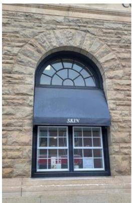
Figure 55: Detail of the side (southeast) elevation of the existing building at 78 Main Street South, showing the arched window opening with radial stone voussoirs (Town of Halton Hills 2025)
